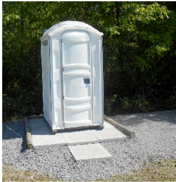
Assembly and installation of new Polyjohn restroom
